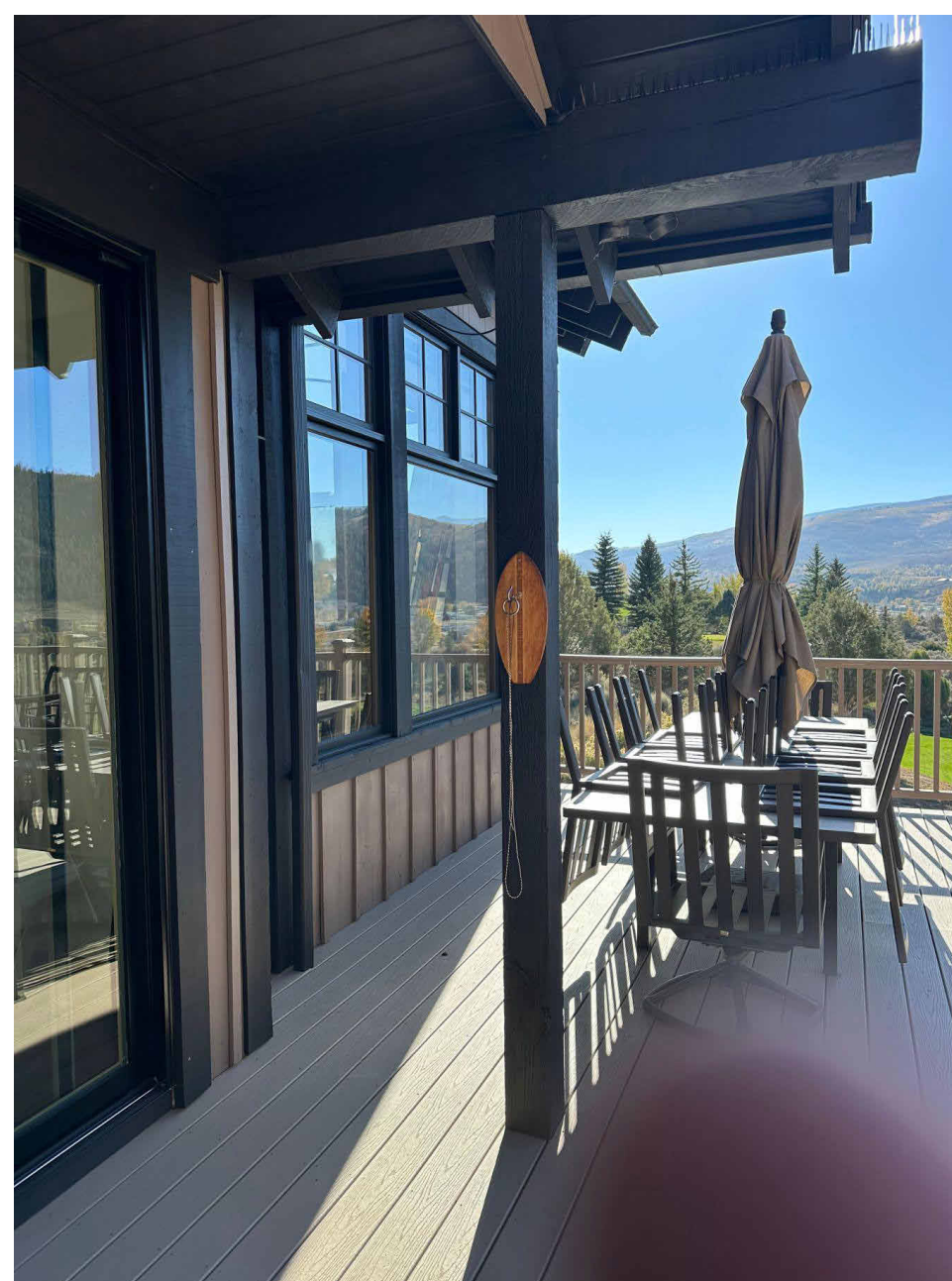
AT DECK LOOKING SOUTH
