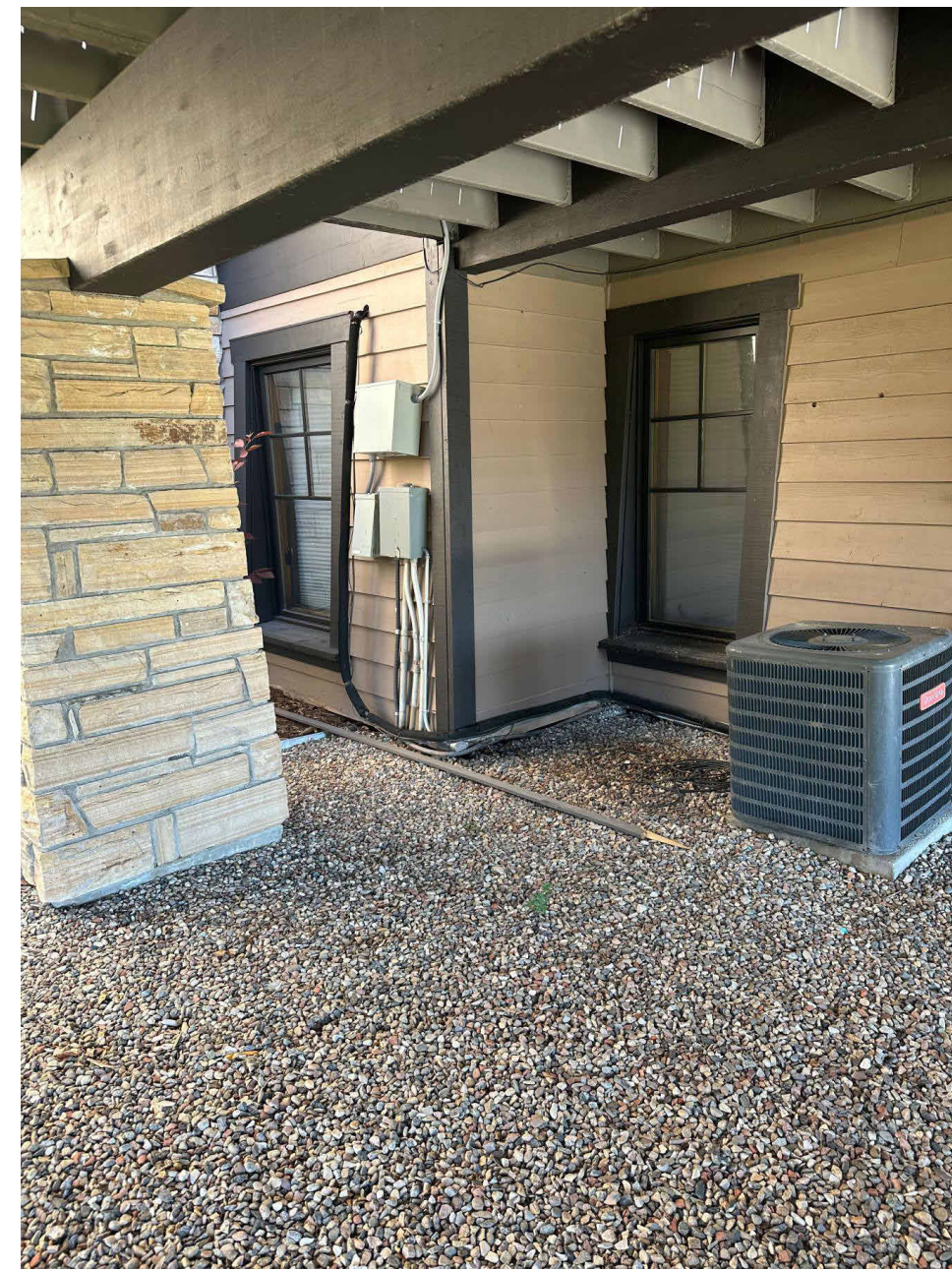
LOOKING NORTH UNDER DECK - AC UNIT TO BE RELOCATED
