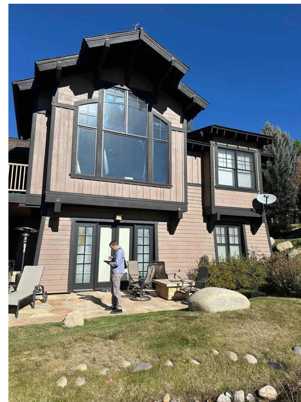
TERRACE PAVERS TO BE PRESERVED
