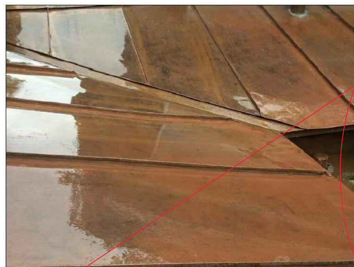
6 PRE-WEATHERED COPPER ROOF
