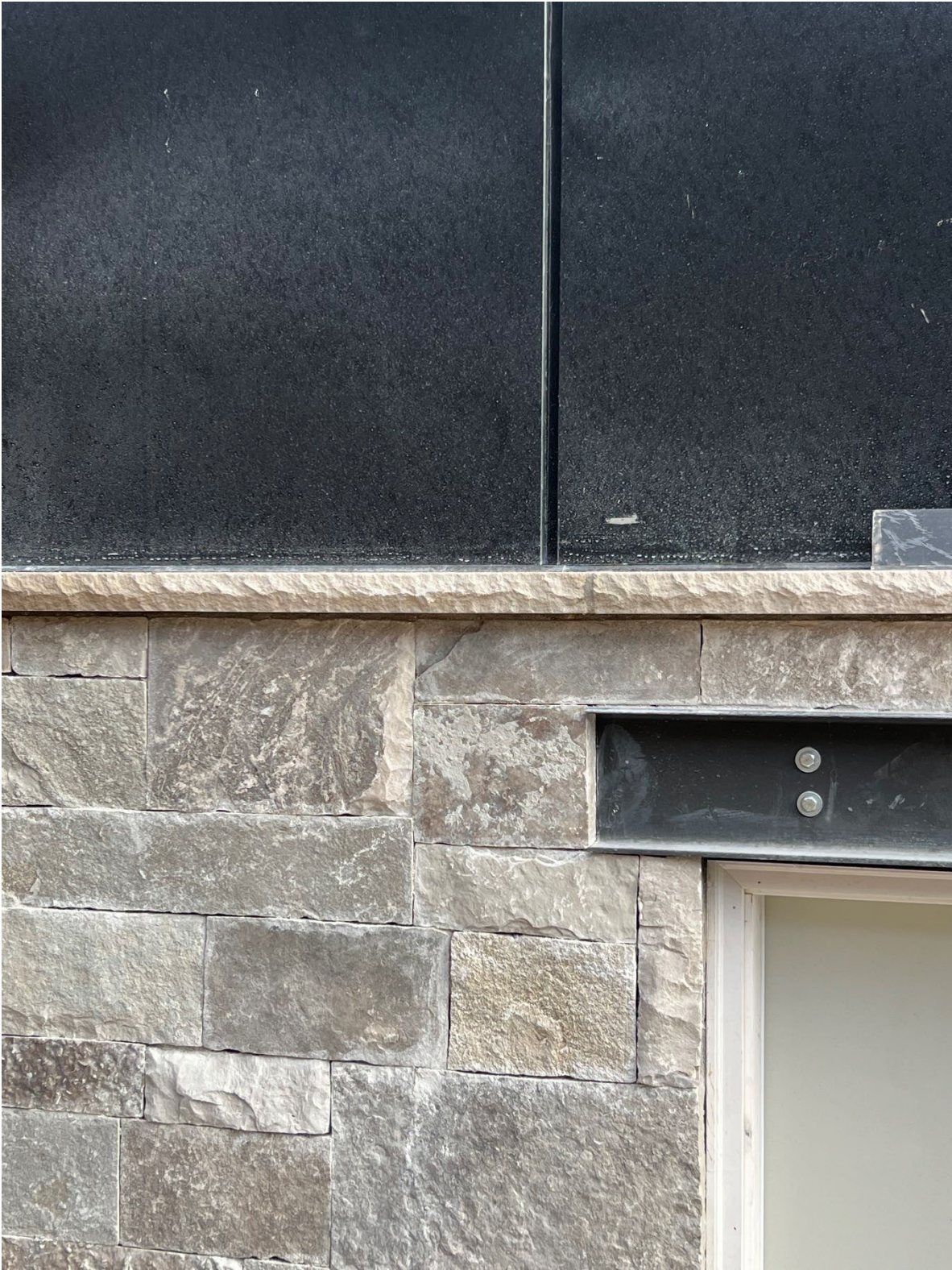
F-4 Break Metal Siding: Black Break Metal paneling shown with transition to stone sill. Panel reveals 3/4"
