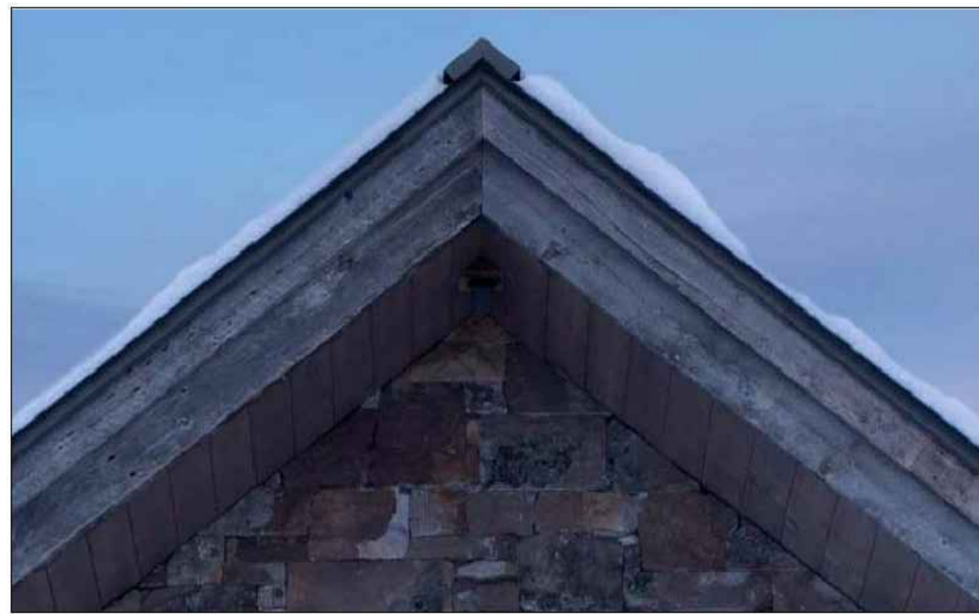
4 WEATHERED FASCIA AND STONE
